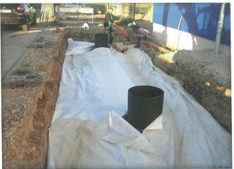
Gravel backfill allows direct seepage and long-term safety at drainage. Single fleece coat only needs to be placed above and on the sides of the tank.
